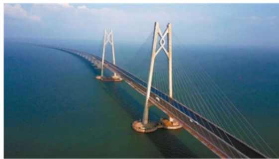
Figure 1. Hong Kong–Zhuhai–Macao Bridge
